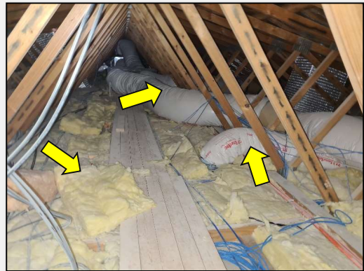
Photo 4: Ground floor, internal, ceiling cavity - SMF-containing insulation batts and insulation to ducting
