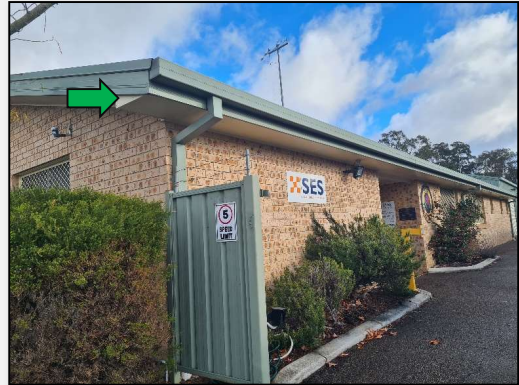
Photo 2: Ground floor, internal, gable ends at eaves end - non-asbestos fibre cement sheeting
