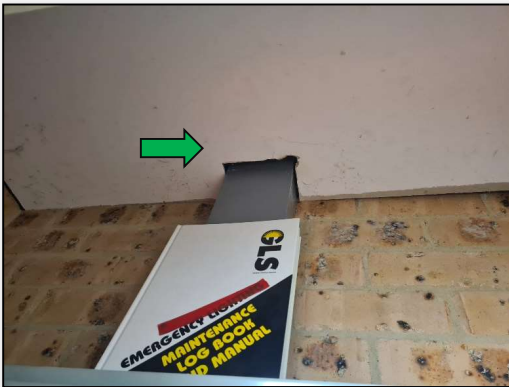
Photo 3: Ground floor, internal, electrical board ceiling - non-asbestos fibre cement sheeting
