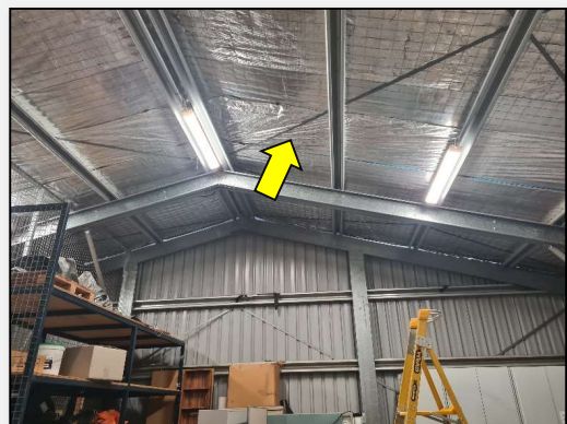
Photo 6: Ground floor, internal, garage ceiling cavity - SMF-containing sarking insulation
