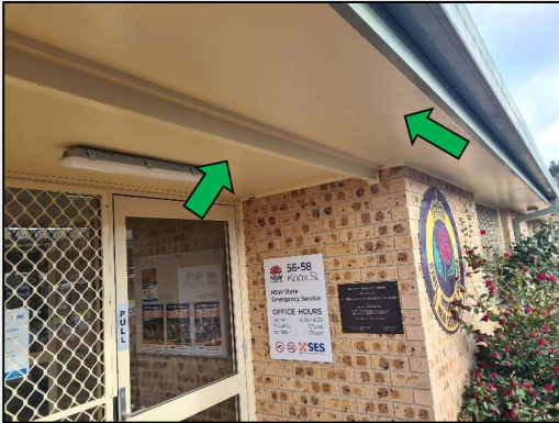
Photo 1: Ground floor, external, eaves linings all sides and entrance awning - presumed negative fibre cement sheeting
